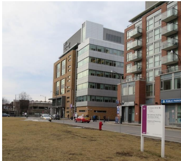
Queen Street Site
